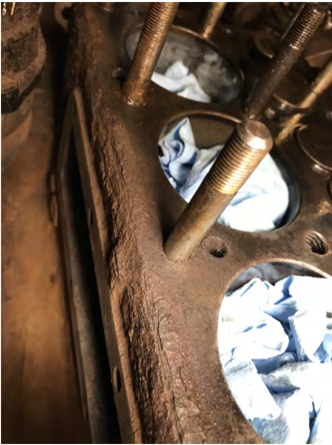
Of concern was starboard side with corrosion - preservation required
