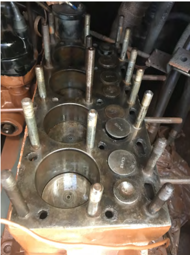
Eleven new studs installed - nylon zip tie used to ensure clear cooling passages
