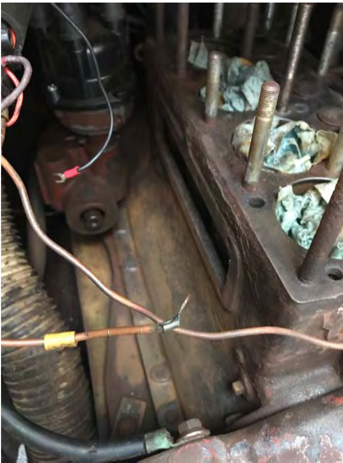
Final engine (starboard) descaling and cleaning
