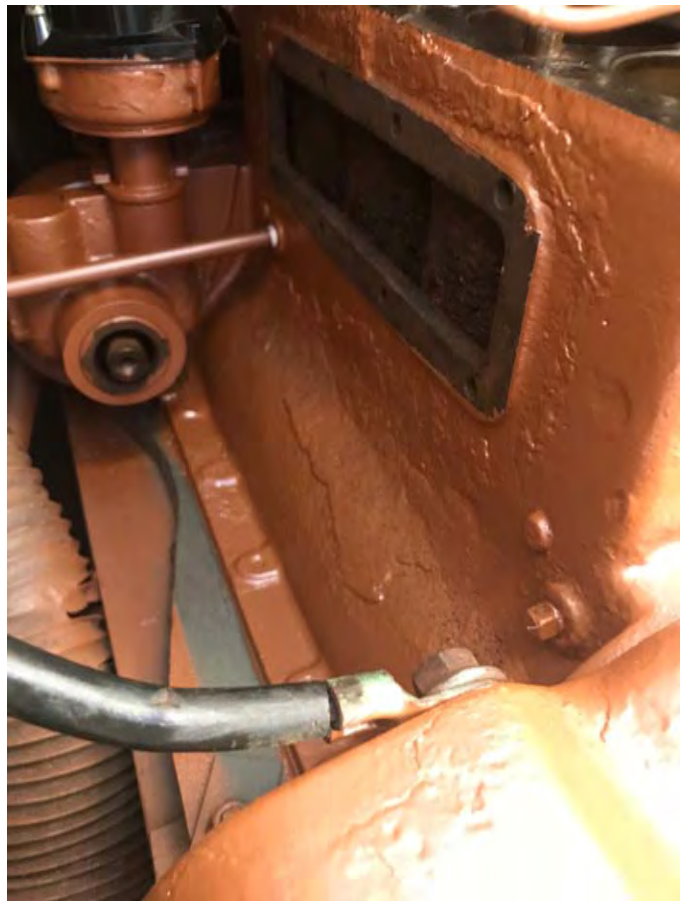
Finishing coat (starboard side)
